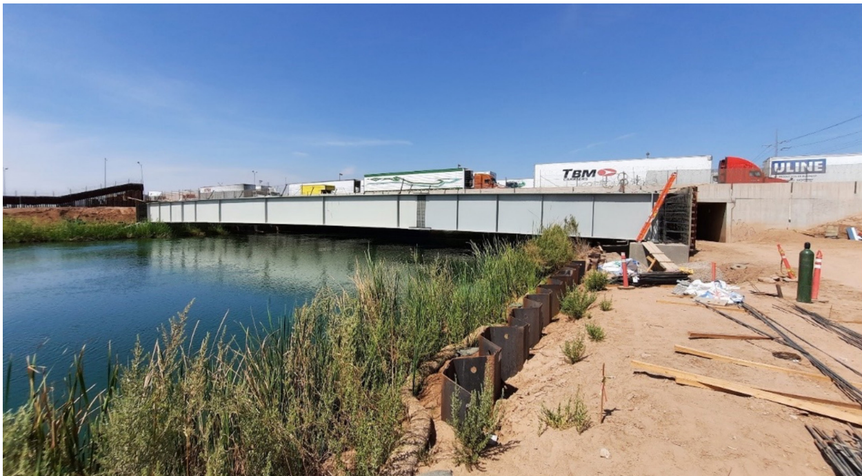
Figure 9. Calexico Bridge Widening
