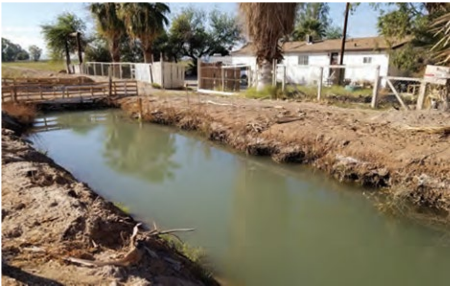
Photo Caption: Unlined, open-air canals provide water for domestic use to rural homes in Imperial County. Image Courtesy: OEHHA
