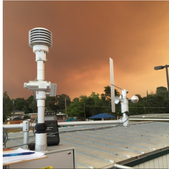
E-BAM PM monitor calibration during Valley Fire.
