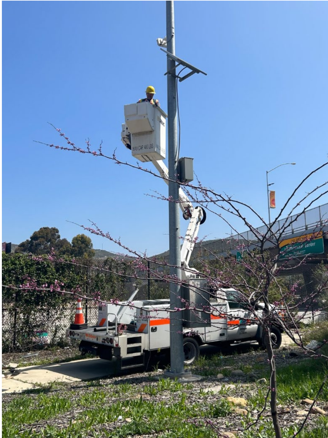
Photo 6: Air Quality Monitor installation near San Ysidro Port of Entry
