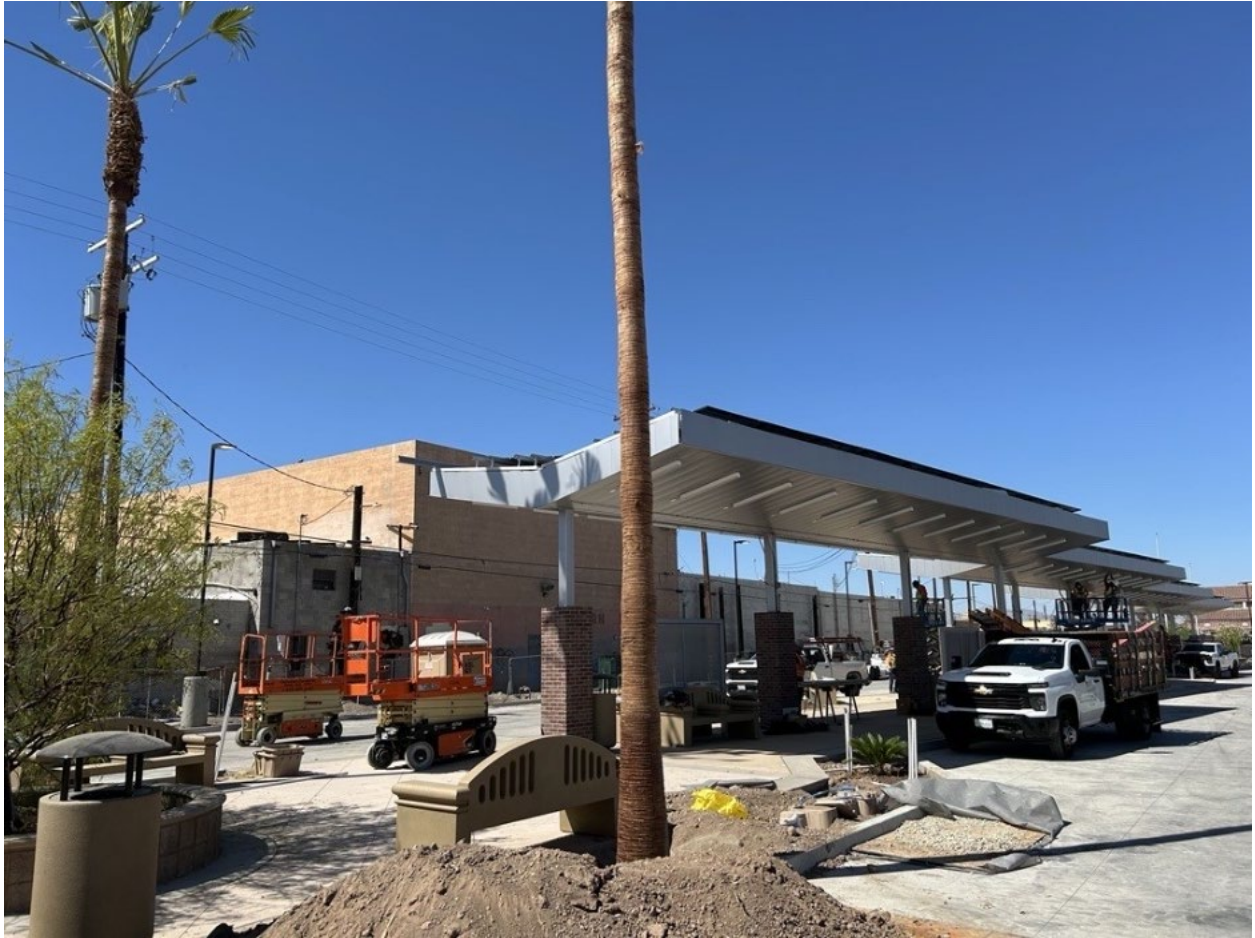
Photo 5: Imperial County Transportation Commission- Intermodal Transit Center in Calexico under construction
