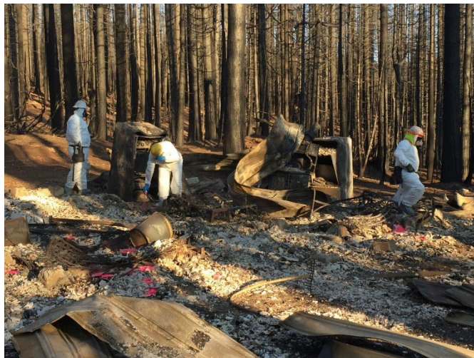
Photo 3: DTSC-led Hazmat crews conducting Phase 1 Assessments/Removals of debris in Plumas County. Photographer unknown.
