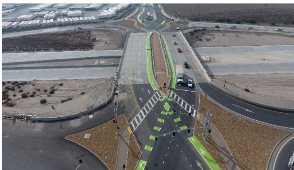
SR 11/Enrico Fermi Diverging Diamond Interchange (DDI), second DDI in the State of California
