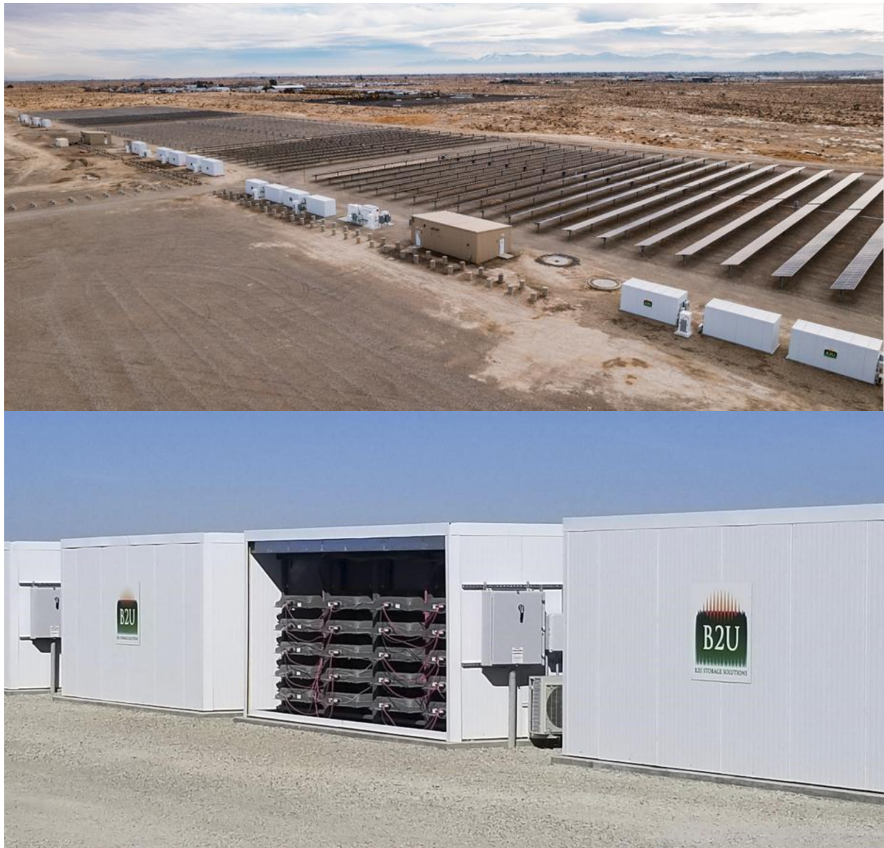
Figure 2: B2U Storage Solutions' storage system at a solar PV field in California. The current operational system capacity is 8MWh and will be increased to 17MWh by Q2 2022. (Photo credit: B2U Storage Solutions)
