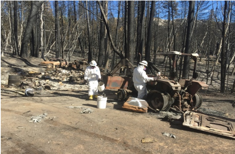
DTSC Hazmat Crews conducting Phase 1 Assessments and removals for the North Complex Fires in Butte and Plumas Counties. Photographer unknown.
