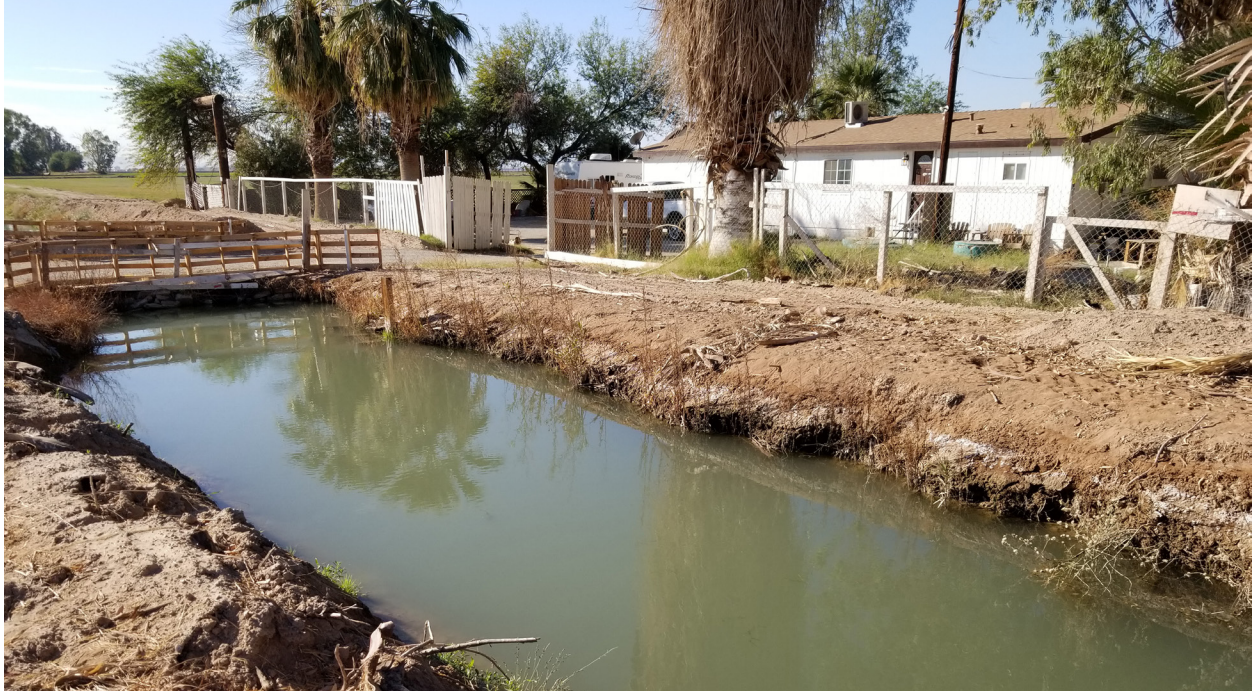
Unlined, open-air canals provide water for domestic use to rural homes in Imperial County. Image Courtesy: OEHHA
