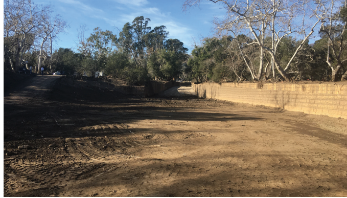
Cleared debris basin.
