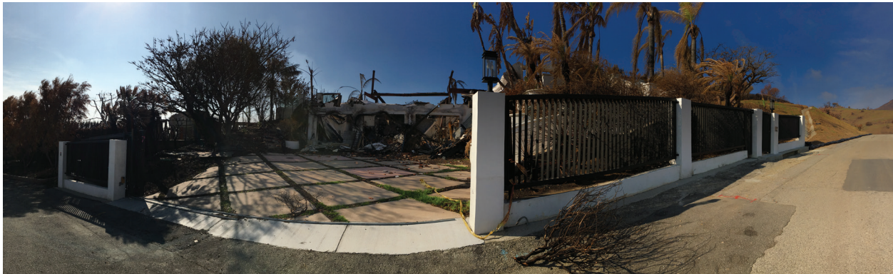
House burned and damaged from Camp Fire.
