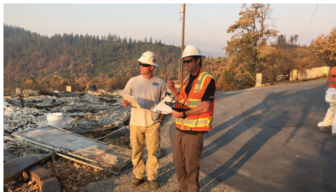
DTSC crews assessing destroyed buildings after the Carr Fire.
