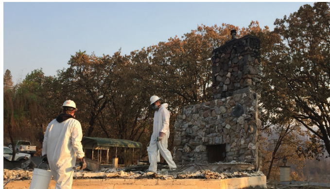
DTSC crews removing household hazardous waste from a home destroyed by the Carr Fire.
