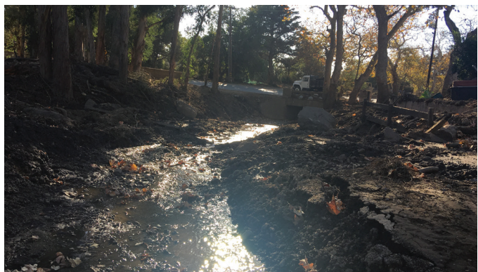
Creek cleared of sediment and debris.
