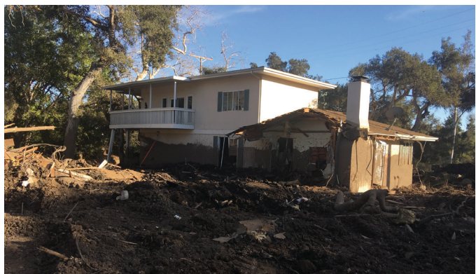
Debris flow damage.
