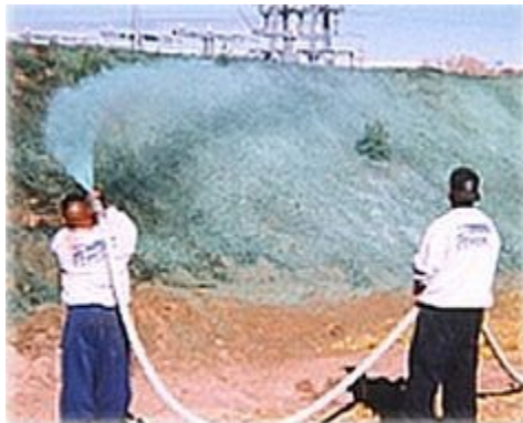
Hydroseeding is a popular technique for applying seeds, fertilizer, and chemical stabilizers in a single application (Source: Terra Firma Industries, 2000)
