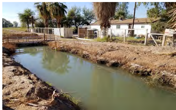
Unlined, open canals provide water for domestic use to rural homes in Imperial County
