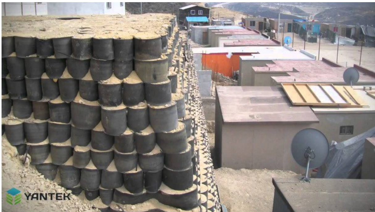
Image 2. Yantek constructed retaining wall and house pad. Source: Yantek.
