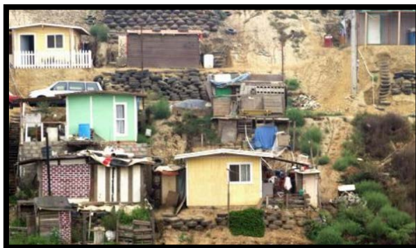
Figure 10 Recent self-constructed housing in newly developed areas in the upper Los Laureles watershed. Note the use of scrap tires for foundations, retaining walls, and stairways. Source: 2009 Waste Tire Study
