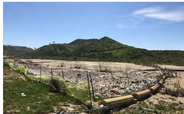
Goat Canyon Lower Trash Boom. Image Courtesy: Chris Peregrin, California Department of Parks and Recreation
