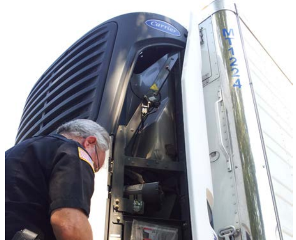
Inspection of diesel-powered transport refrigeration unit
