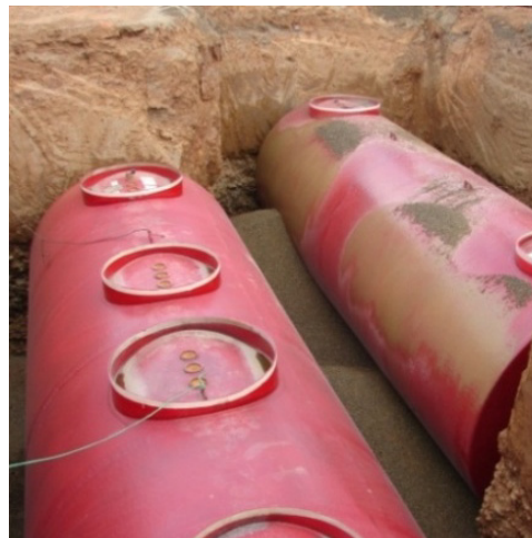
Inspection of underground storage tank
