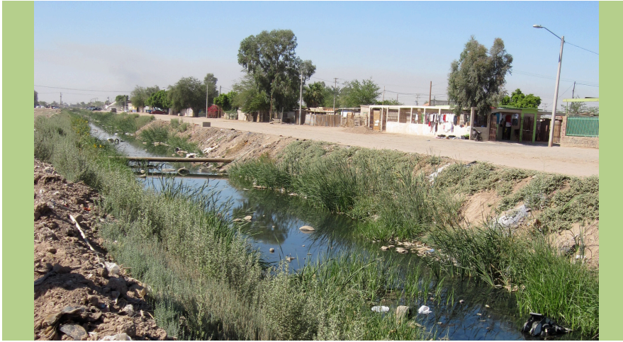
Open drainage ditch in Mexicali.
